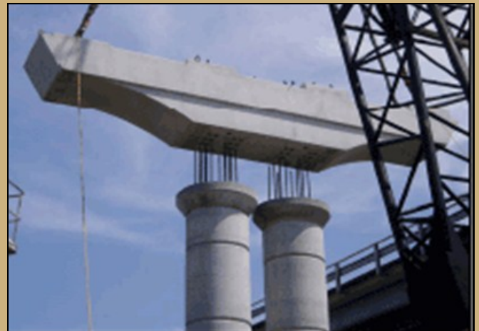
Connection for a prefabricated bridge element
