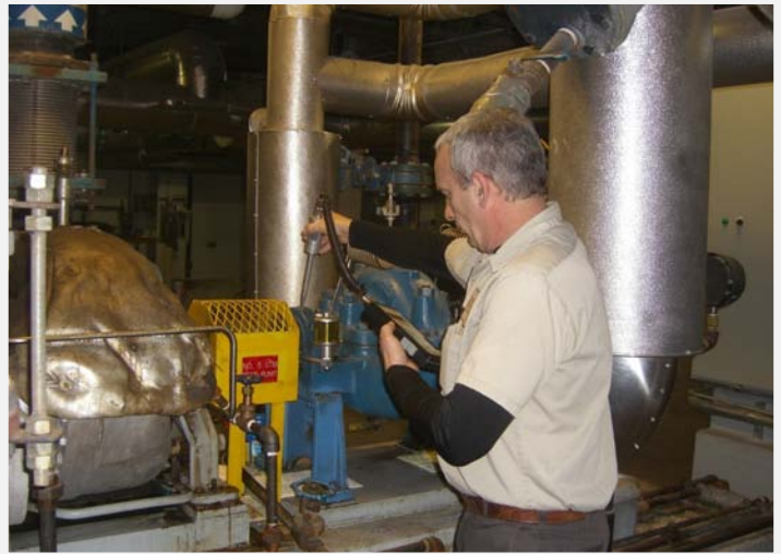
Pictured is one of our power plant operators, Tom Maida, performing a vibration check on the steam turbine driven feed pump. Our skilled personnel are trained in all aspects of pump maintenance and rebuilding.
