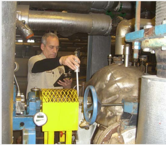
Pictured is one of our power plant operators, Tom Maida, performing a vibration check on the steam turbine driven feed pump. Our skilled personnel are trained in all aspects of pump maintenance and rebuilding.
