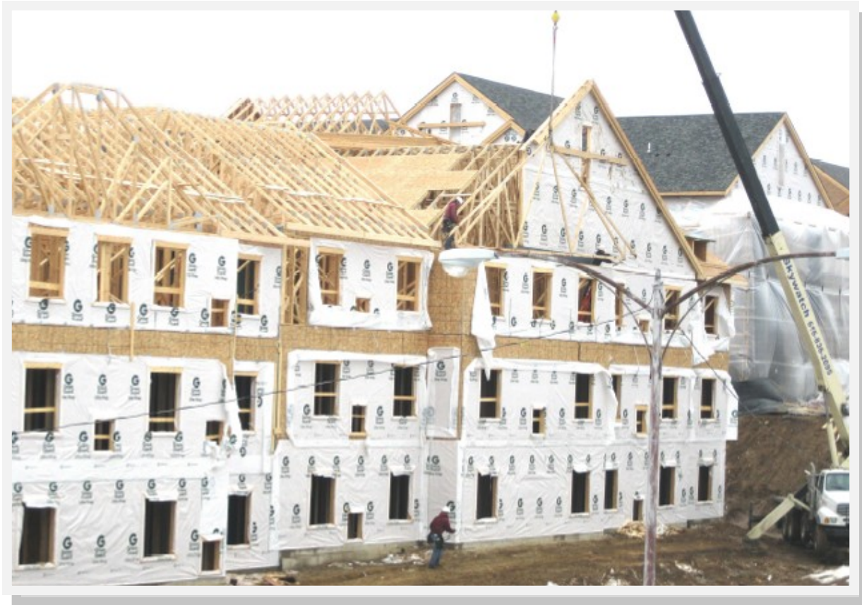
Western View Apartments: Roof Being Installed
