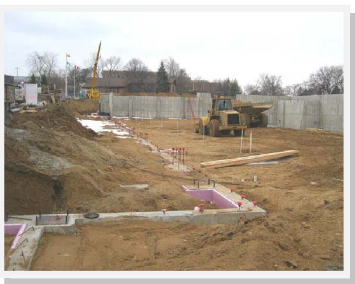
The New Sangren Hall: Footings on the Southside of the building
