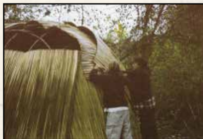
Figure 12. Assembling a pek-ye-gan (wigwam), a mat covered winter house, 2001.
