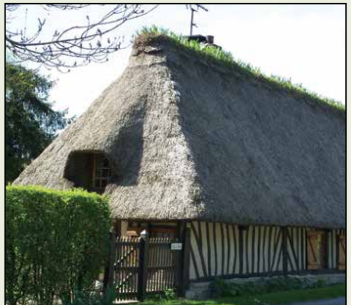
Figure 31. This house found in Normandy, France was built using the poteaux sur sole method.
