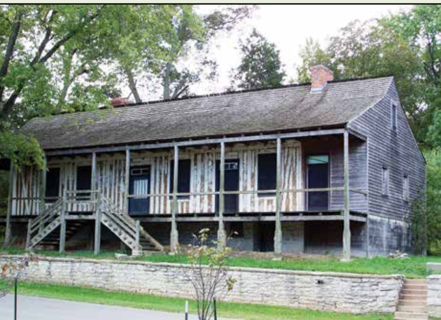
Figure 37. The Janis-Ziegler House in Ste. Genevieve was built with an attached gallery raised above ground level.
