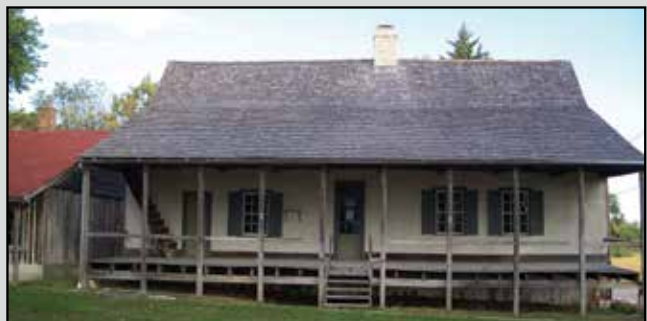
Figure 3. The Bauvais-Amoureux House, located in Ste. Genevieve, was built using the poteaux en terre construction method and exhibits a double-hipped roof and front gallery.
