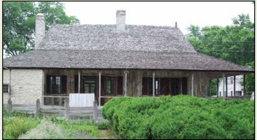
Figure 30. The Bolduc House in Ste. Genevieve, Missouri exhibits a double-hipped roof and gallery.
