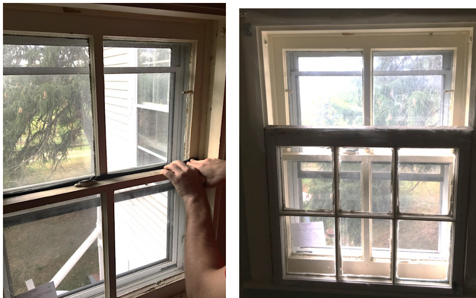
Figure 7: Standalone window baseline (left); standalone retrofitted window installed (right)
