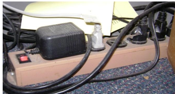
4. Potential fire hazard from outdated power strips in offices.
